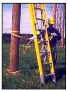
2d. Pull both strap cinches until both sides are snug. Be sure both loops are tight against the underside of the fifth rung of the ladder.
